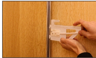
Insert STR002-HG into STR002 on both sides and fix.
