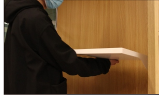
Insert the STR002- HR of the installed wooden laminate into STR002 and fix it.
