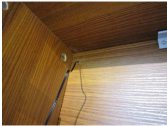
Step I: Cut a 4mm hole at the back of the cabinet.
