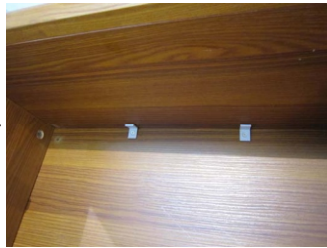
Step II: Screw the mounting clips at the corner.
